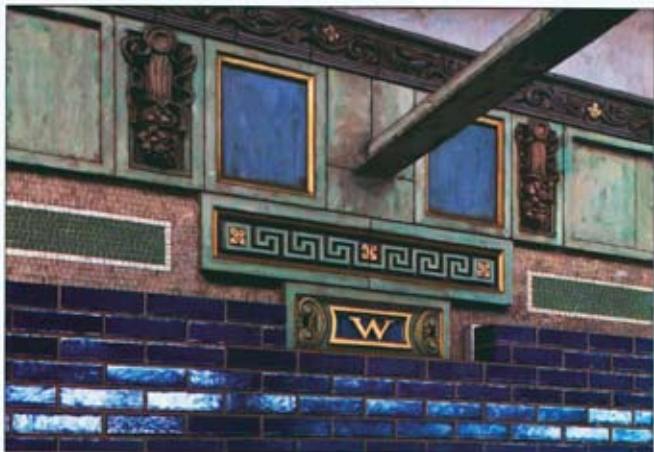
Wall Street - Steel Beam
